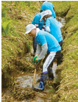
Employee volunteers removing mud from side ditches
